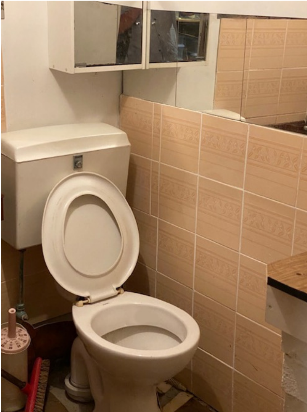
spa bathroom toilet
