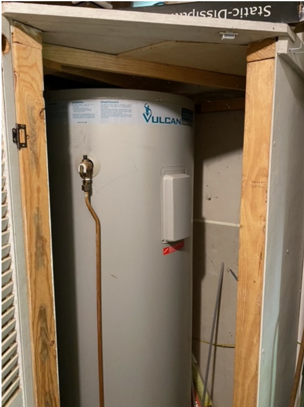
HWS built-in cupboard
